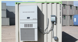
100 Amp sub panel with exterior outlet & j-box to inside
